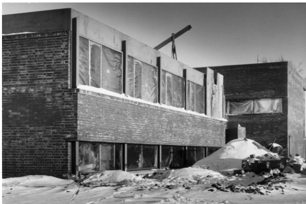
New Township Offices under construction, Feb. 1963. EHS06606
