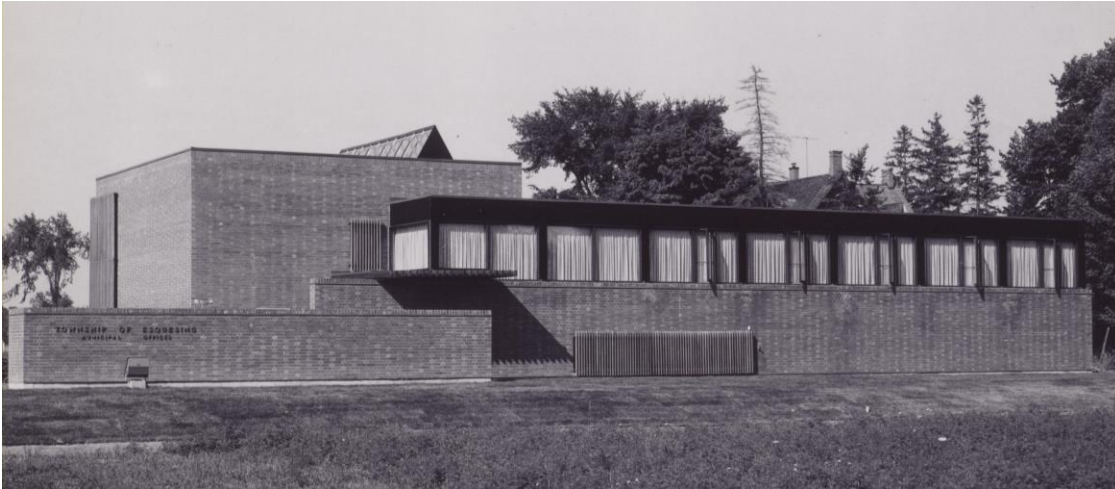
The completed Esquesing Township Office, August 1963
