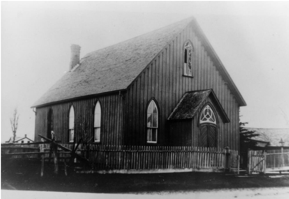
St. John's Anglican Church , 10966 Trafalgar Road, Stewarttown.
