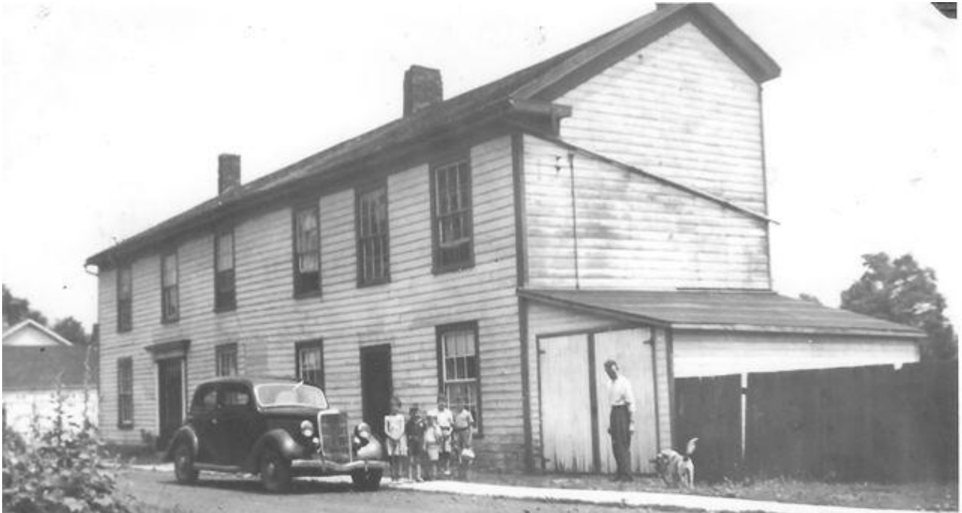
Former Limehouse Hotel 1948
