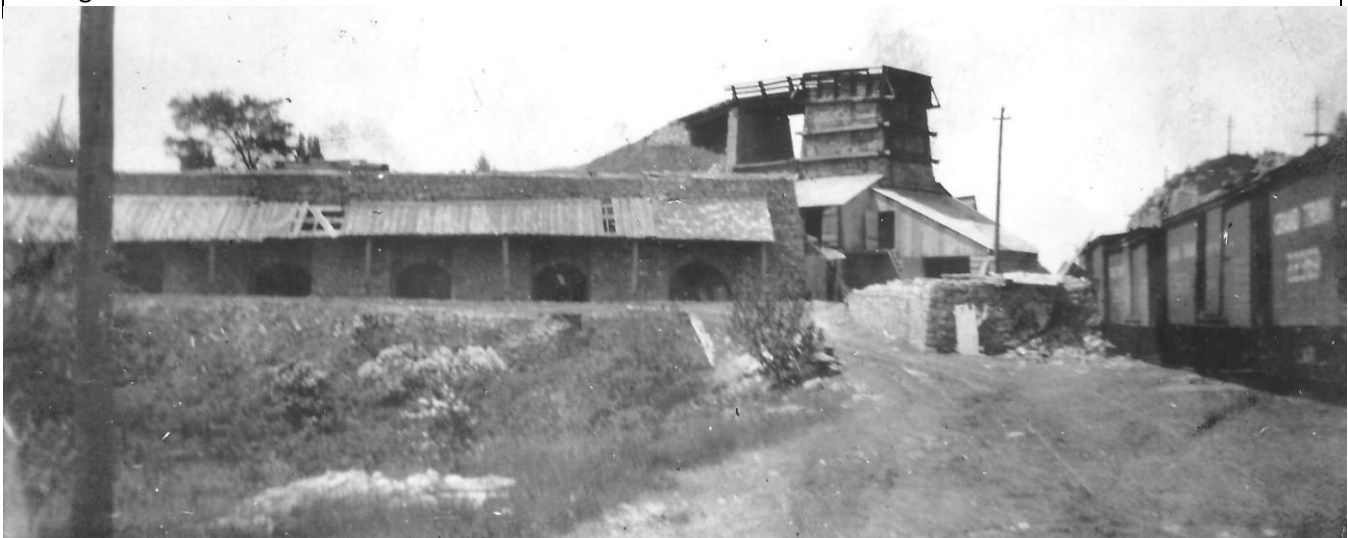
A view of the set kilns with protective lean-to roof, the draw kiln above them and box cars on the railway siding. C. 1891
